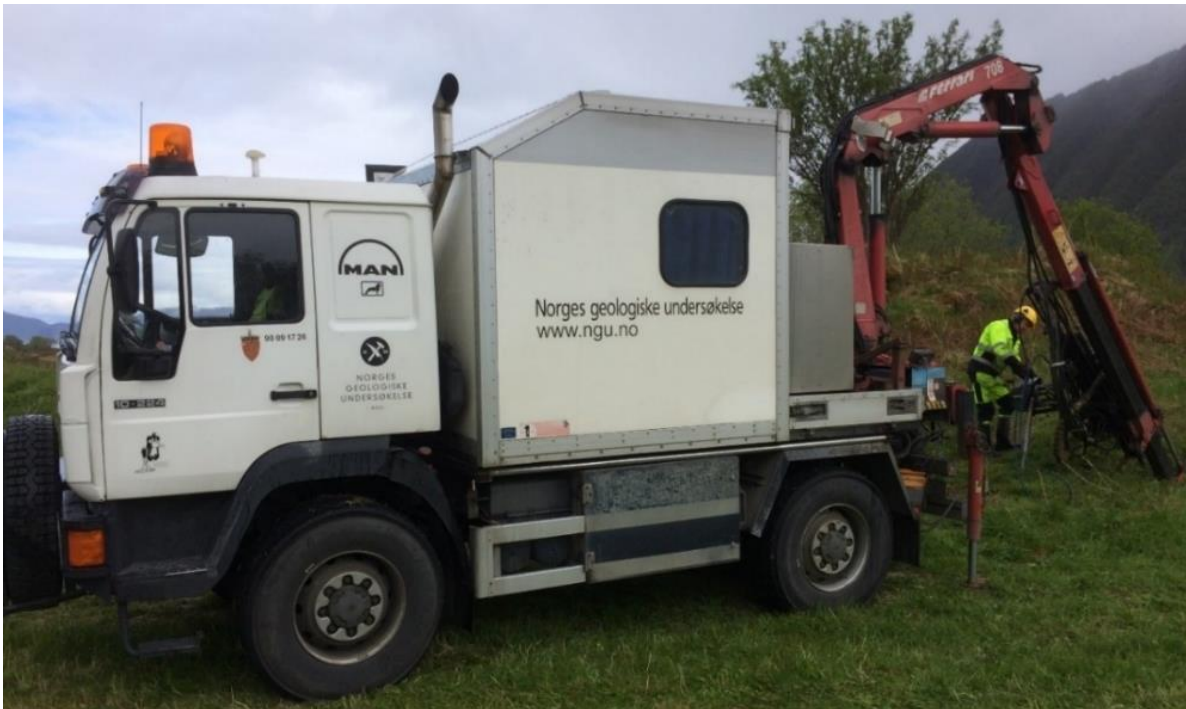
Figure 4.7: NGUs truck mounted drilling gear in operation.
