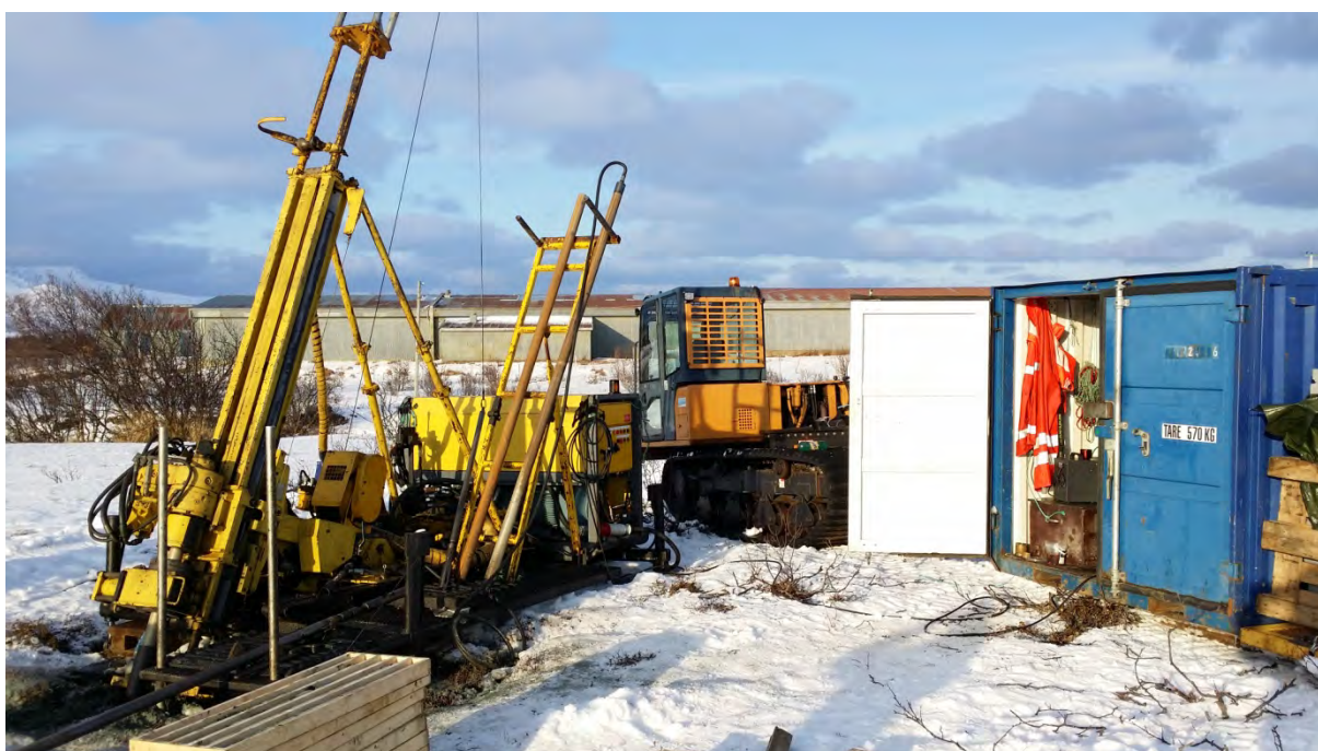
Figure 8.3. Drilling rig Diamec U-4 APC at location BH 4.
