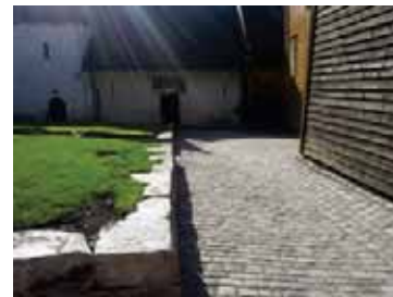
Permeable pavement and adjustment of the terrain surface stimulates local infiltration of storm water runoff. On the left hand side, green swales are visible that actively store and infiltrate rainwater. Photo: Johannes de Beer, Geological Survey of Norway.
