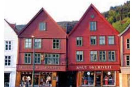
Subsidence in the archaeological deposits underneath Bryggen has caused severe structural damages to the historical wooden buildings. Photo: Johannes de Beer, Geological Survey of Norway.
