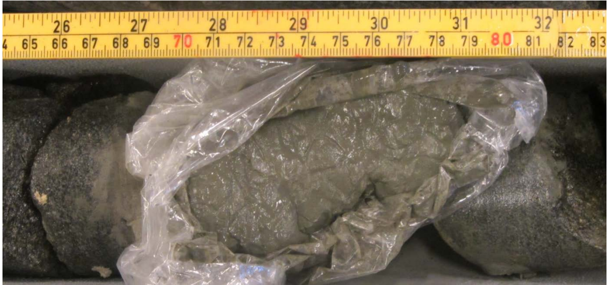
Figure 3. Clay zone at ca. 60.77 with 2-3 cm thickness. This clay zone is located at end of a ca. 10 cm zone of crushed rock. The clay is well developed and mainly contains fine grained material, therefore this zone is regarded as the main zone of movement, and is possibly a sliding plane.
