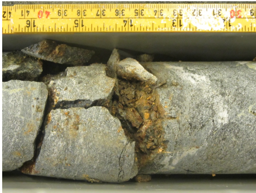
Figure 6. Narrow zone of crushed rock that has rusty colour at ca. 167.35 m, indicating water flow along the fracture/zone.
