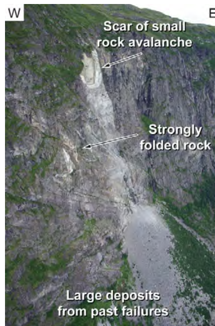
Figure 83: Photograph of the Jimdalen rock slope: the scar and deposits of past rockfalls and a small rock avalanche are visible, but no open cracks or structures delimiting a large unstable rock slope are visible.
