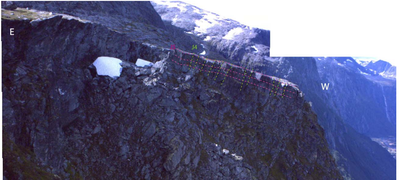
Figure 11: view of the upper site with the 6 discontinuity sets.
