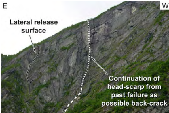
Figure 80: Photograph of the potential instability Alvikhornet 3 that is delimited by a possible back-crack, a poorly developed lateral release surface and a basal sliding surface probably formed by exfoliation.
