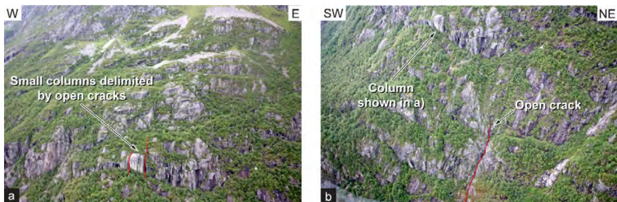
Figure 69: Photographs of the Mjølvafjellet rock slope: open vertical cracks affect the vegetated rock slope and locally delimit small columns that might lead to rockfalls.
