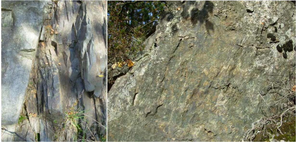
Figure 53. Left: western border of 5 m wide, steep NE-SW basaltic dyke at field point “Erlandstuveien_3”; note the high frequency of vertical NE-SW joints within the dyke; right: the north-dipping striated fault observed at field point “Erlandstuveien_4”; (field points are located on Figure 51).
