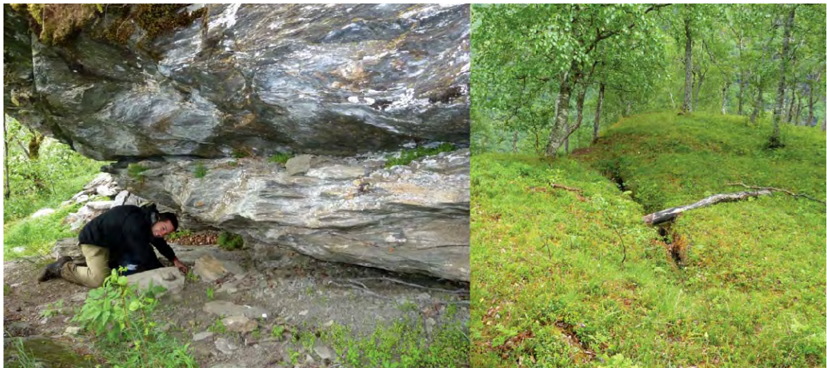
Figure 67. Probable sliding plane at block 1 and an open fracture at the surface.
