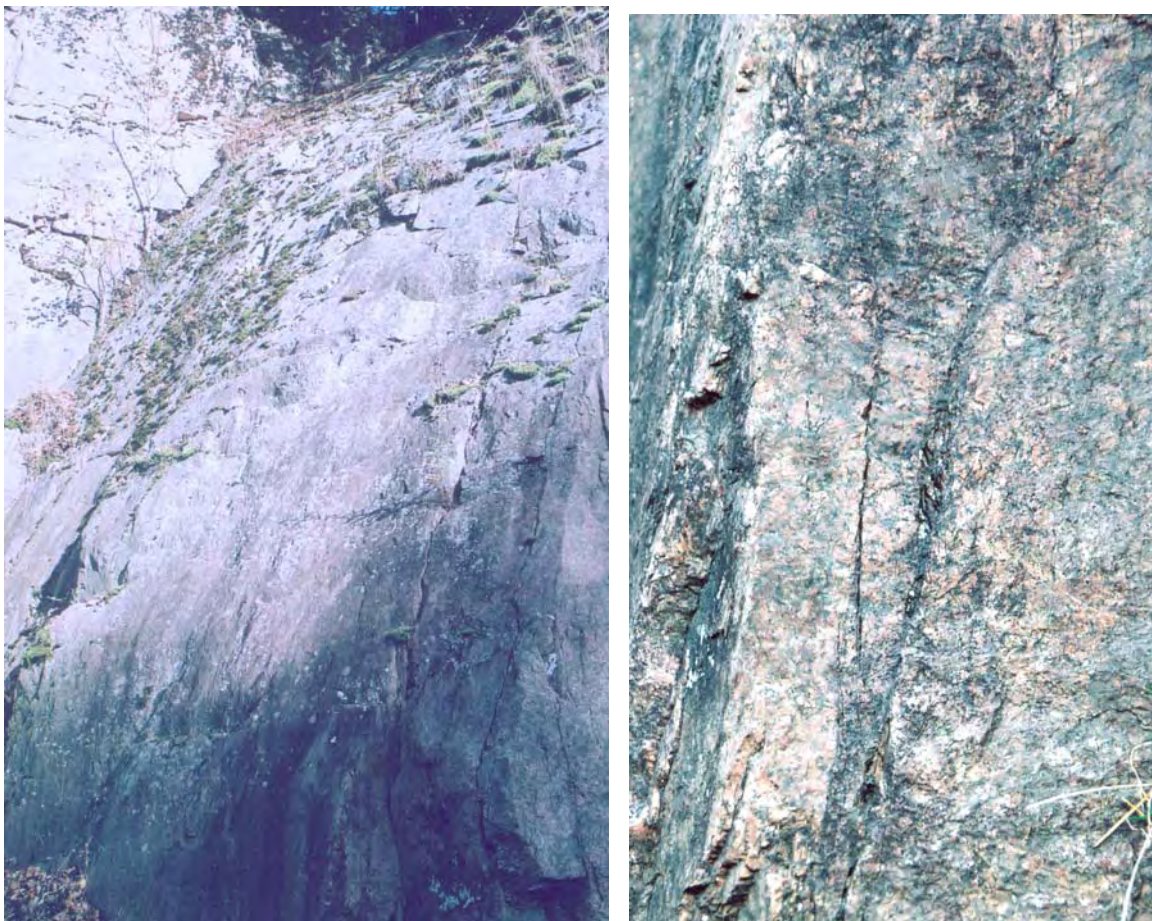
Figure 26. Left, large N185 striking dip-slip normal fault at site 29 (Granheim). Right, a side view of the fault plane, with well-developed shear fractures.
