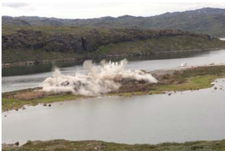
Figure 2 The first blasting of the Seqi deposit (source, MINELCO web page)
