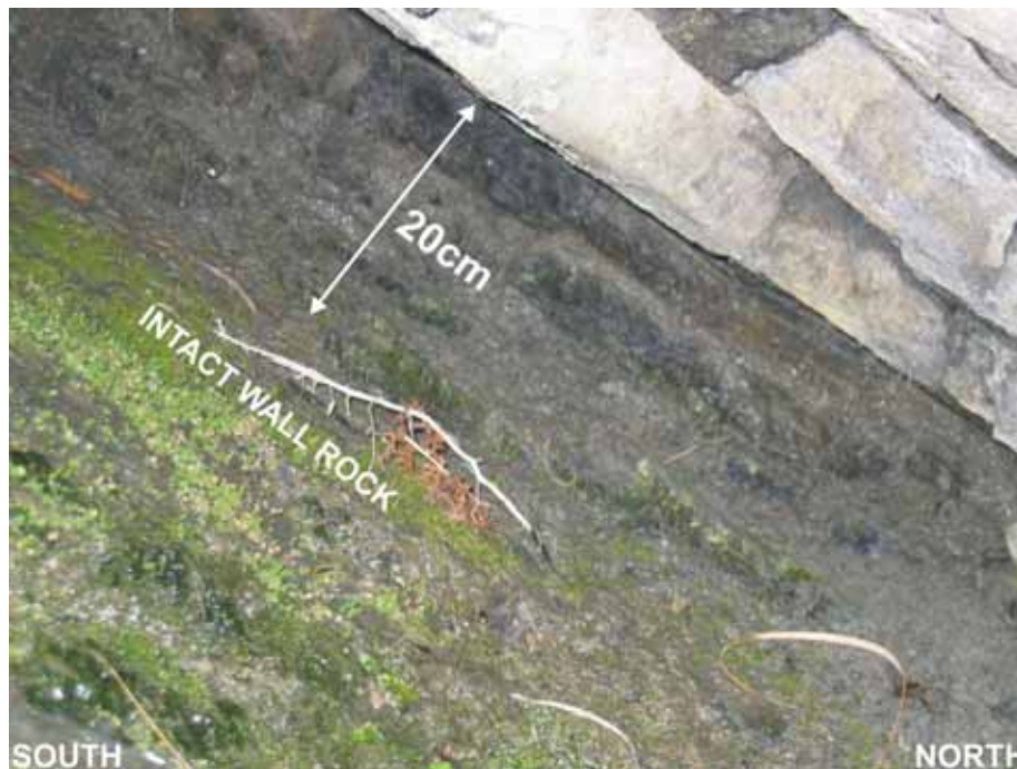
Figure 20: Fault gouge developed at Site 7b. The gouge is up to 20cm thick but is discontinuous along the fault plane. The contacts with the intact wall-rock are very sharp.
