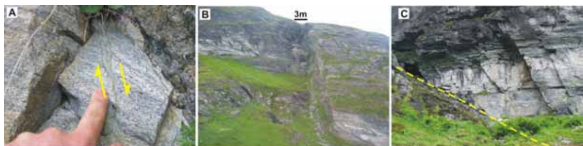
Figure 17: A-Extensional fractures are a reactivation of north-south trending epidotised cataclastic faults. B- View of the back-crack fracture. C-Extensional fractures in the potential failure block in the hanging wall to the low-angle sliding plane (in dashed yellow line).
