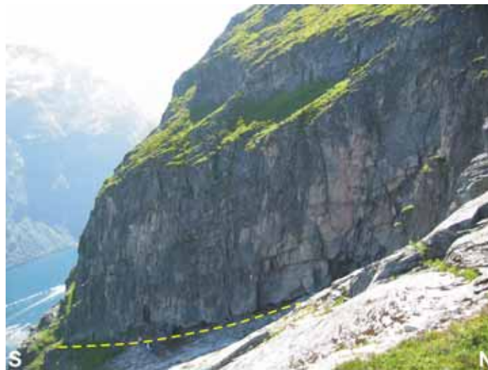
Figure 33: Structures observed in outcrop at Site 12. The dashed line is at the base of the postulated unstable block is interpreted as a low-angle sliding plane. The complex and dense suite of fractures and joints within the unstable block appears to stop at the base of the block, suggesting that their formation is related to the movement on the basal shear plane.
