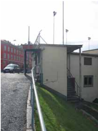
Figure 34. The area around Bislett stadium is subsiding between 1.5 and 2.0 mm/yr. Two PS have subsidence rate of 5 mm/yr, however these are located on the corner of a structure supported by a wooden post. It is most likely that this post is slowly deteriorating, leading to a slow collapse of the roof.
