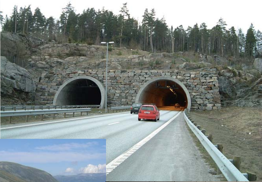
Brick wall made from local gneiss on highway E6, Vestby municipality, Akershus.
