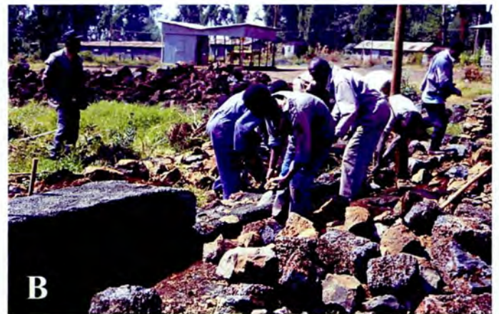
Figure 34 A) Quarry in columnar basalt, Ambo. B) Building wall of vesicular basalt.
