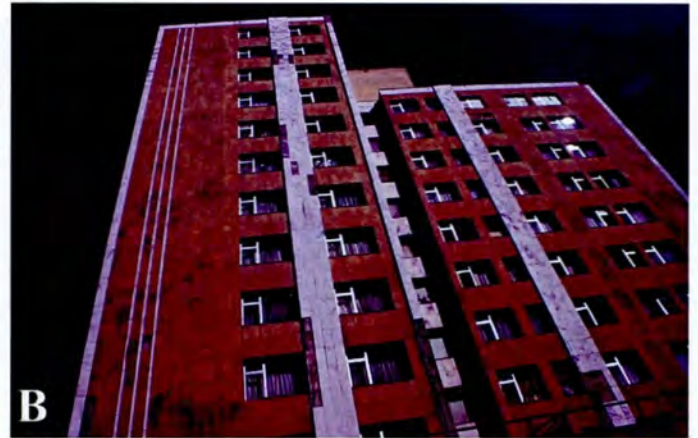
Figure 26 (above) A) Limestone beds in the Hakimgara quarry, Harar. B) The Hakimgara limestone used as facade cladding in Addis Ababa, combined with stripes of the Daleti marble.
