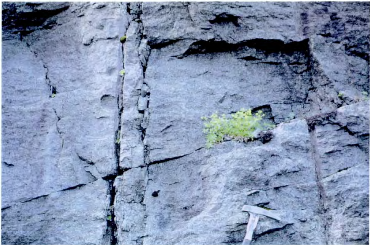
Fig. 4.6.1 Reverse-faulted offset drillholes in Proterozoic granulite gneisses, along the road to Roan, south of Beskelandsfjorden (NE of Roan). Photograph taken looking SSW.
