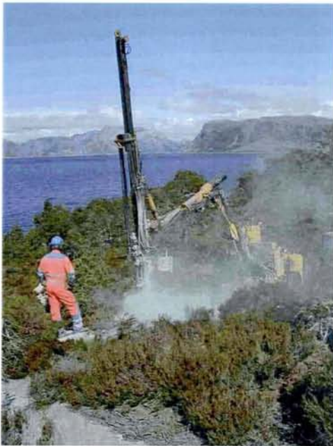
Figure 3. The drill site at Gulestø.
