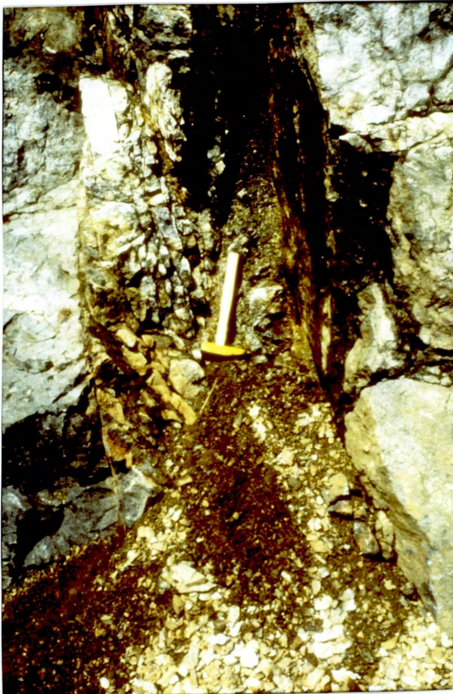
Figure 20. (A) 'Zone A' (where the hammer is placed) and 'zone B' (left of hammer) of vertical fault in gneiss at Sandvika, near Askvoll in Sunnfjord. (B) Zone A (two < 25 cm zones of breccia - deeply eroded) and zone B in quartzite along the Eikefjorden fault near Alnakken, Sunnfjord. Note the dense network of short fractures (locally > 100 f/m; zone B). The stick is 1 meter long. (C) Close up of the photograph in Fig. 20B, showing details of zone B.
