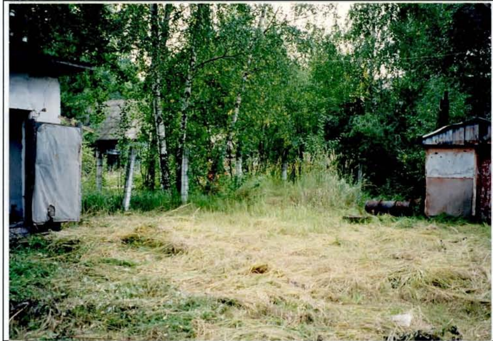
Photograph 5: Drums visible outside one of the buildings forming part of the chemical storage area. Sample Lit II-1 containing 1,2 dichloroethane was taken from one of these drums.
