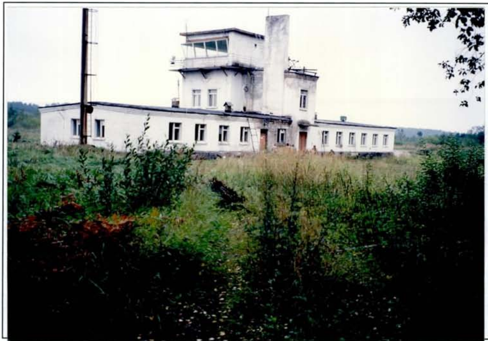
Photograph 8: The main building at the radar facility in the centre of the airfield.
