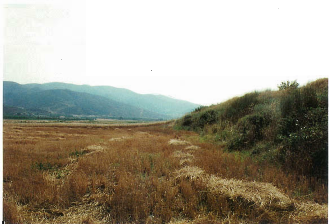
Fig. 3. Flood protection works.
