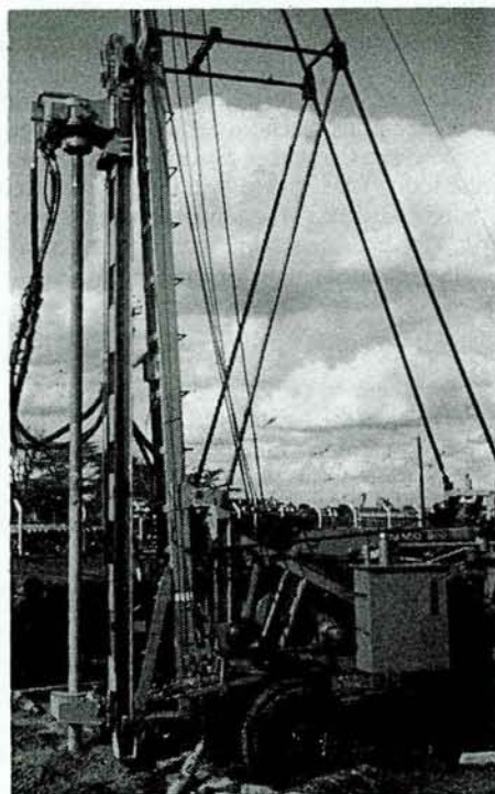
A Dando-800 percussion rig with rotary attachment working in Kenya.
