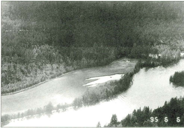
Fig. 5. Erosion scar by the 200-year flood in the Østerdalen valley, Norway. The protectional structures along the river have caused turbulence on the floodplain and a large trench was carved out by the flood (Photo by J. Bogen, 1995).
