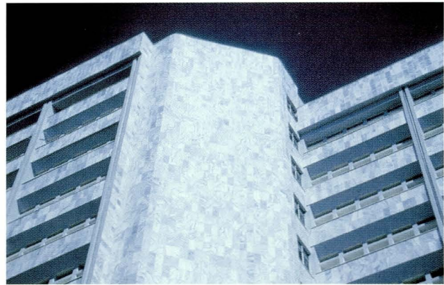
Fig. 2. The Daleti marble (Wellega) cladding the facades of a modern building in Addis Ababa.
