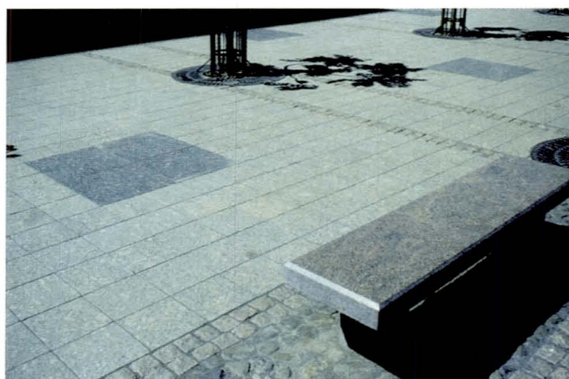
Fig. 6. Polished surface of the variegated Babile granite (right) and flamed and honed tiles of the porphyritic Anger Guten granite (left). Hotel Sheraton, Addis Ababa.
