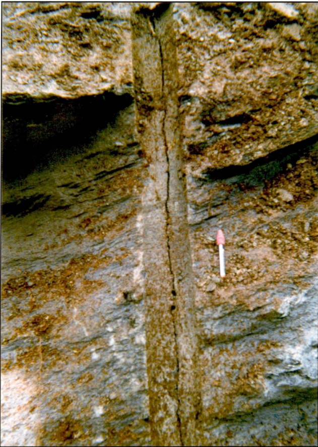
Fig. 3. A particularly well developed, continuous axial fracture in a drill-hole penetrating mica schists. Locality along a new section of the E39 road, currently under construction, 1.5 km east of Børsa, southwest of Trondheim.
