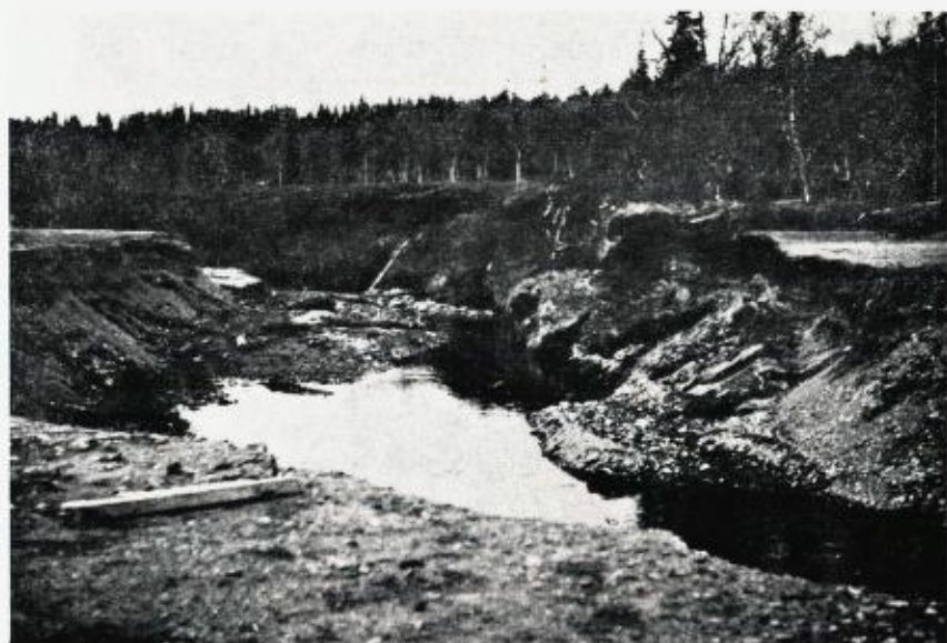
Fig. 8. Limingdalselvens nedskjæring inntil 2/6 1954 ved utløpet i Limingen. The deepening of the Limingdal stream until 2/6 1954 at its outlet in Limingen.
