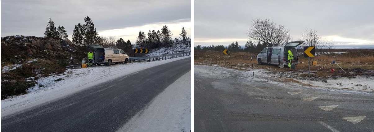
Figure 8. Logging in Bh1 (left) and Bh2 (right). Jøstølen, Smøla, Nov. 2019.
