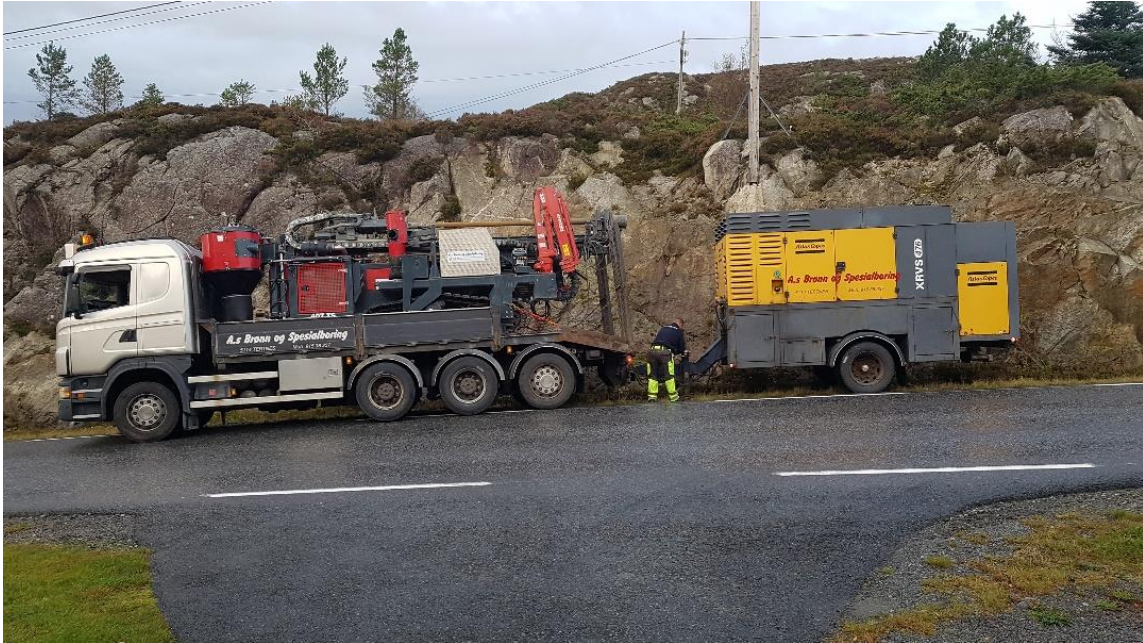
Figure 108. Reopening Bh2 by AS Brønn og Spesialboring.
