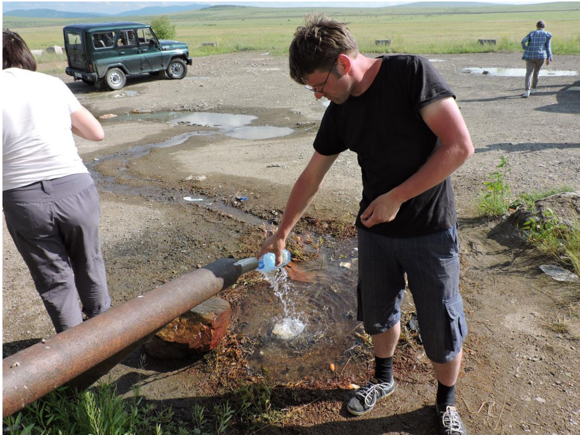
Figure 5.2. Bazanovskii borehole discharge pipe (photo by David Banks).
