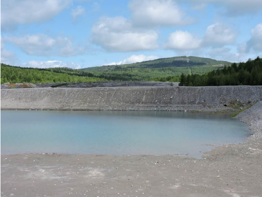
Figure 4.6. Poned mine water on the lower tailings level at Novii Akatui, looking north. The dam at the foot of the middle level can be seen at the rear of the pond (Photo by David Banks)
