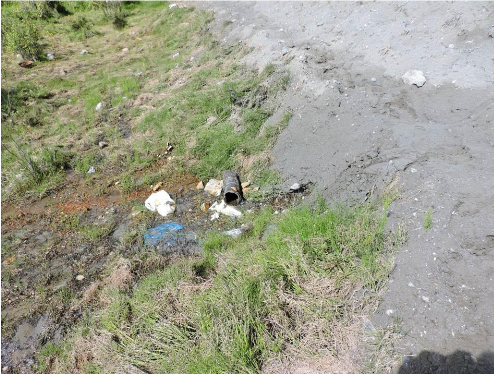
Figure 4.7. Seepage of water from foot of dam at base of lower tailings level at Novii Akatui (pH 6.7, +289 mV). (Photo by David Banks)
