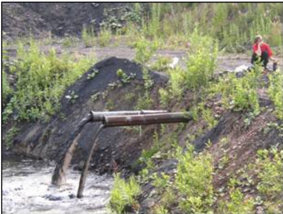
Figure 10.13. Active dewatering of Konyukhtinskaya mine shaft (Xa119)
