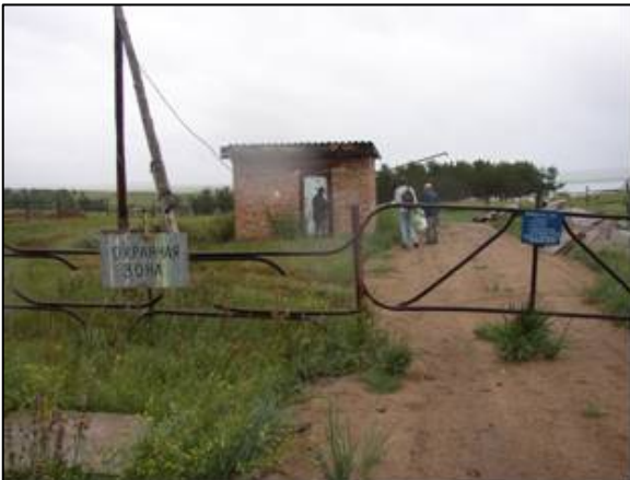
Figure 10.3. Borehole house at Lake Shira kurort (Xa104)
