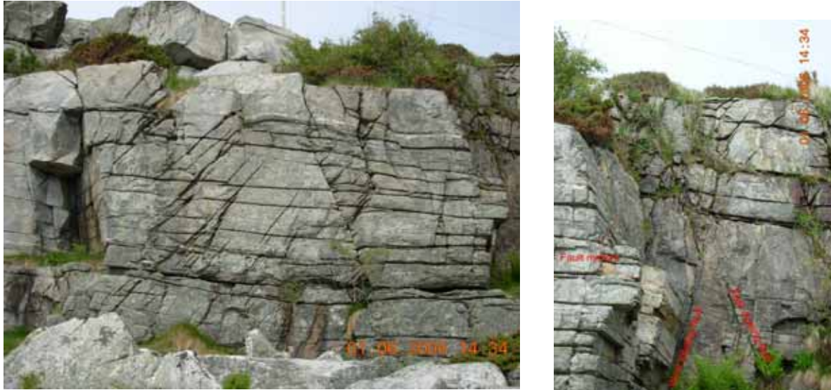
Figure 6.26. View to the N of spectacular extensional structures trending NNE-SSW (site 22); left: network of west dipping extensional fractures; right: normal fault zone.
