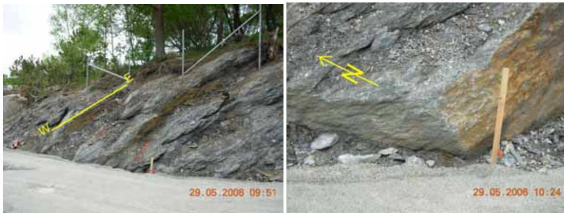
Figure 6.6. Site 1: left, large E-W joints; right, NNW-SSE and E-W joints, probably conjugate system of joints.
