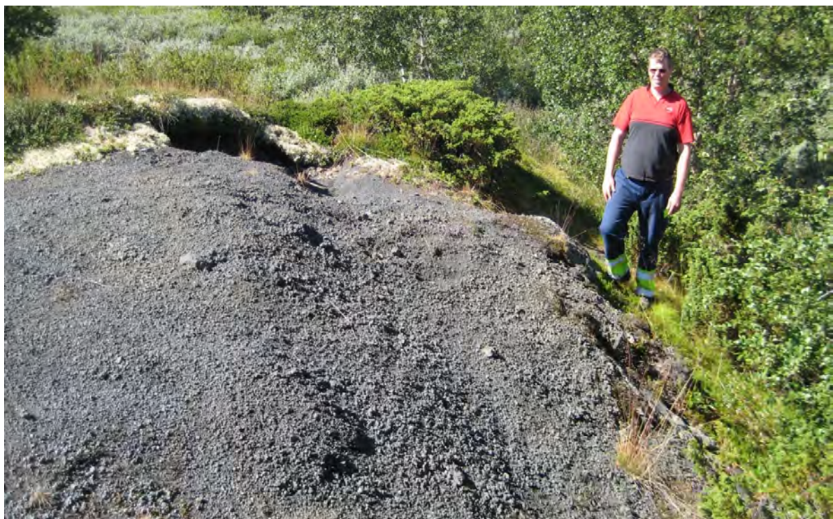
Figure 8.5. Ustaoset locality, showing the deeply weathered gneiss; sample numbers 108513 and -14.
